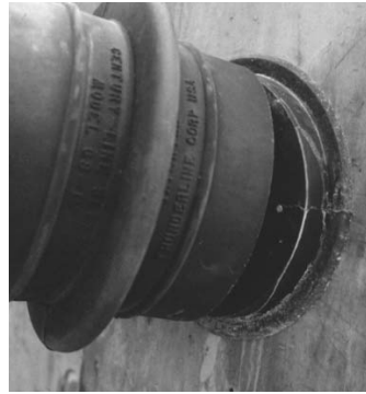
3. Place the Century-Line® Sleeve on the end cap. When field cutting non standard CS sleeve lengths, the sleeve and endcaps total length should be one-fourth (1/4") longer than the thickness of the wall.
