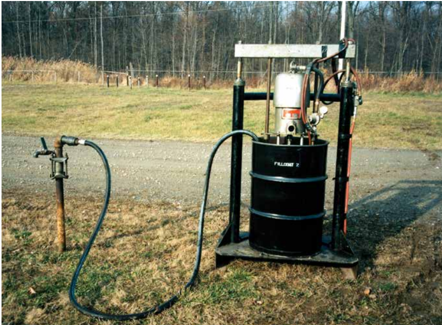
Fill-Coat #2 being pumped by air-driven mastic pump from 55-gallon drums into the casing vent.
